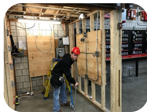
Electrical Sophomore Student "Cade Genard" fabricating an EMT field bend
